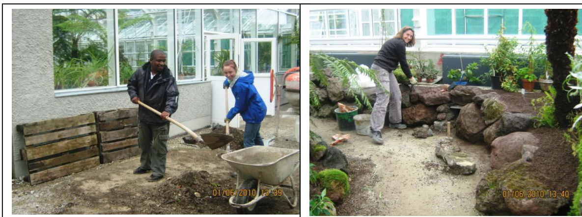
Figure 4: Landscaping works in the Tree Fern house
